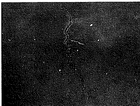
Photo 32 - There are some splits and cracks in the tennis court
