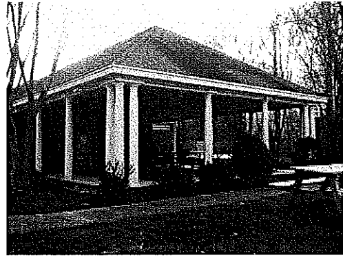
Photo 20 - View of covered patio showing columns, vinyl soffit and trim
