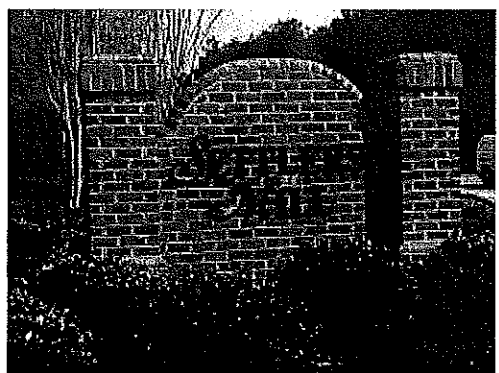
Photo 12 - Entrance monument is in good overall condition
