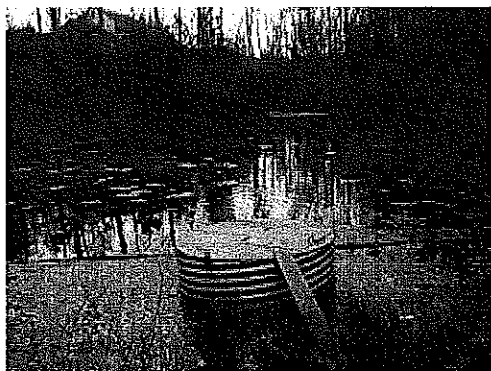
Photo 15 - View of BMP from the earth dam overlooking the spillway - debris should be removed regularly
