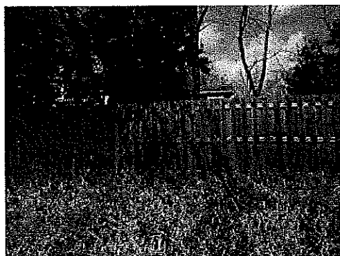
Photo 6 - View of perimeter fence
