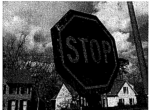
Photo 11 - Several traffic signs are in poor condition
