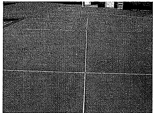
Photo 28 - View of concrete deck
