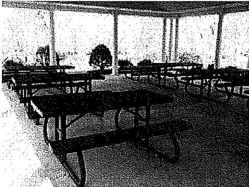
Photo 40 - Metal picnic tables are in fair overall condition
